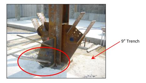
Figure 7: Foundation braced frame connection issues
