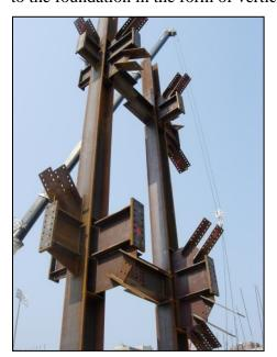
**Figure 6: Connection construction photo**
